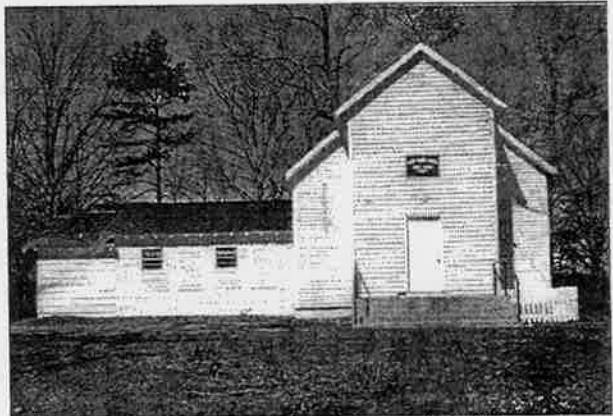
Craigs Chapel (Loudon County) was built in 1896. This view clearly shows the late 19th century school that was moved from nearby and attached by 1940. Center for Historic Preservation.
